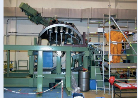
Band saw cutting at Kahl Nuclear Power Test Plant
