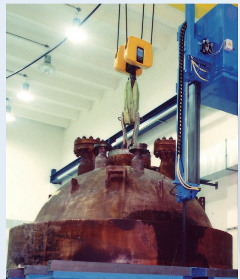
Band saw being used to dismantle large components
