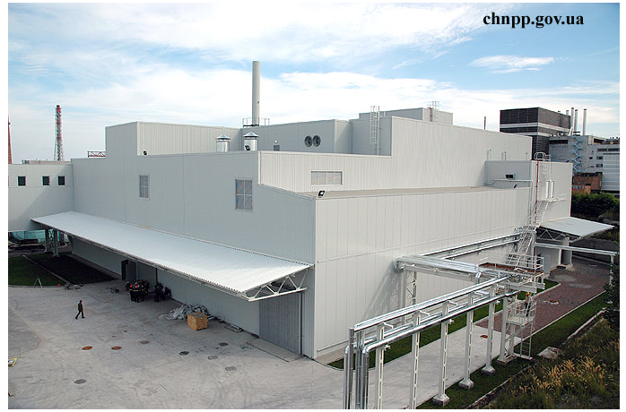
Figure 4: Waste treatment facility
